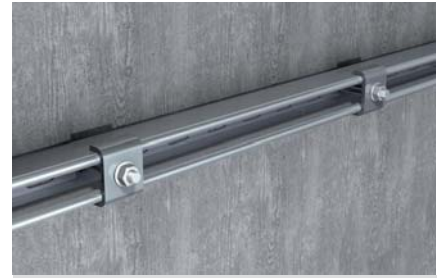
Channel installation at wall
