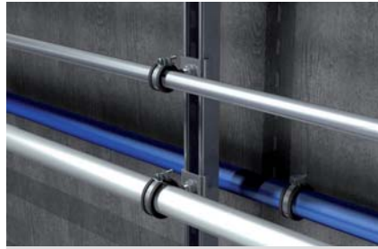
Lateral pipe mounting at channel
