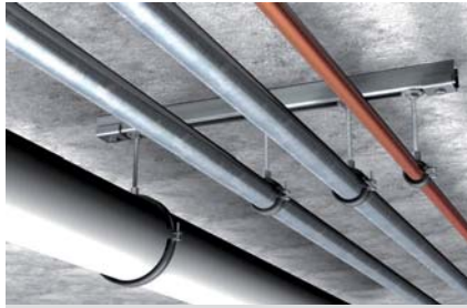
Light, suspended pipelines
