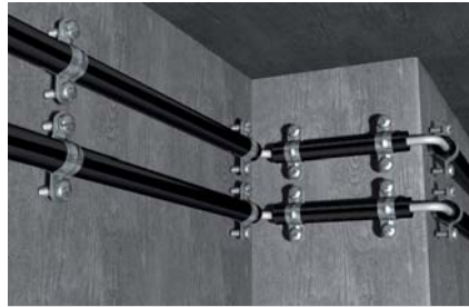
Fixing steel armoured conduits
