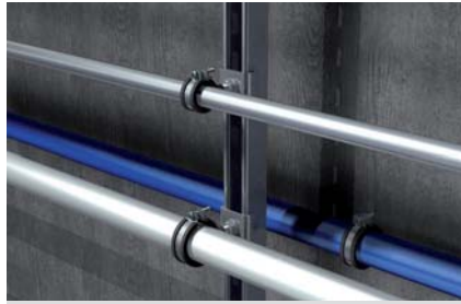
Lateral pipe mounting at channel
