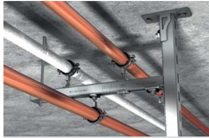
Cantilever construction with channel
