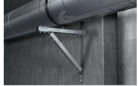
Spiral airtight duct on cantilever
