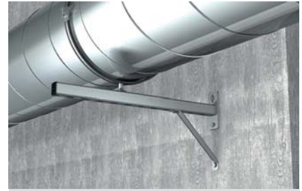
Ventilating pipe fixing at the wall
