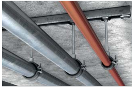
Pipe fixing with channel
