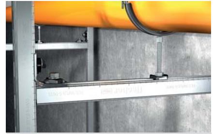
Pipe fixing on frame construction
