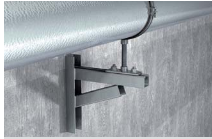
Upright pipe on cantilever arm
