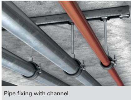
Horizontal pipe fixing
