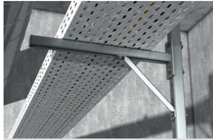
Cable tray on cantilever construction
