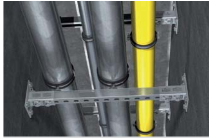
Pipe installation in escape route
