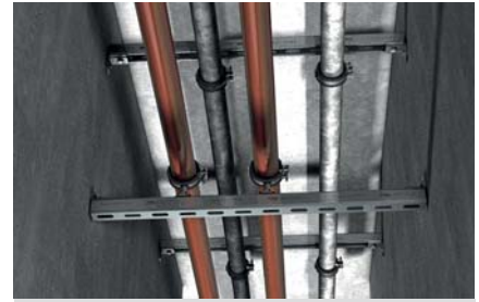
Pipe fixing in a corridor
