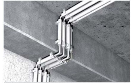
Fixing plastic insulating conduits
