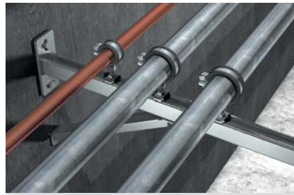
Pipe fixing at the wall
