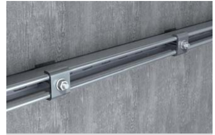
Channel installation at wall
